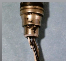
External oil contamination
